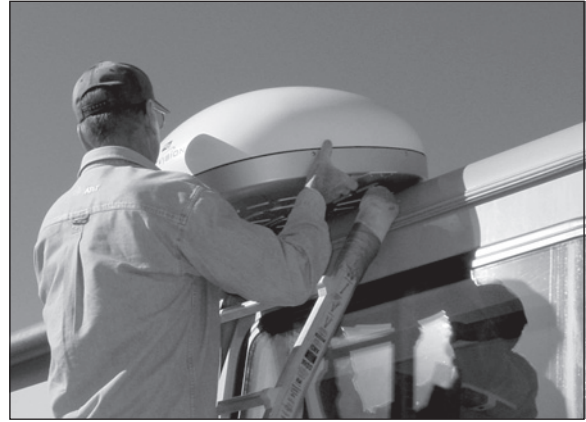
Figure 5 Carrying Antenna to Roof
