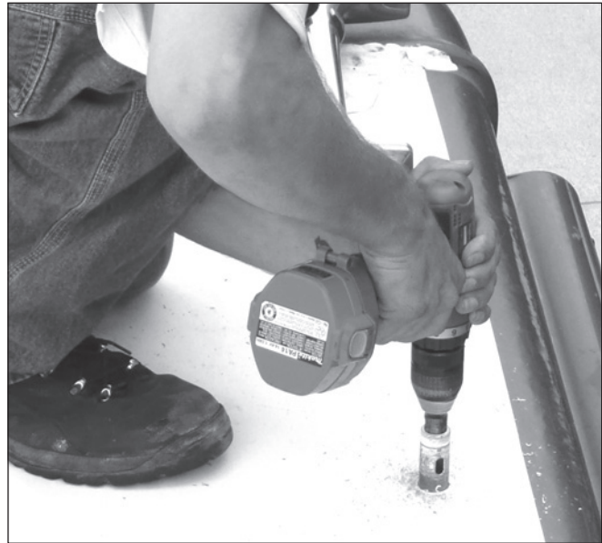
Figure 11 Drilling the Cable Access Hole
